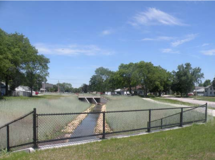
New Dry Run looking from 5th Ave to 4th Ave SW
